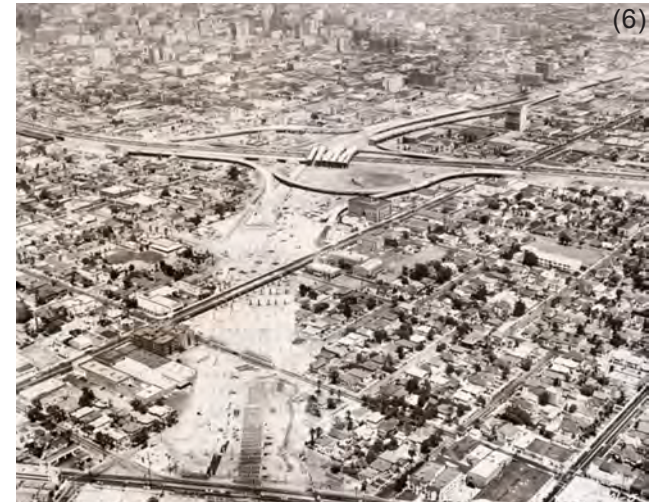
Construction of the East LA Freeway Interchange
