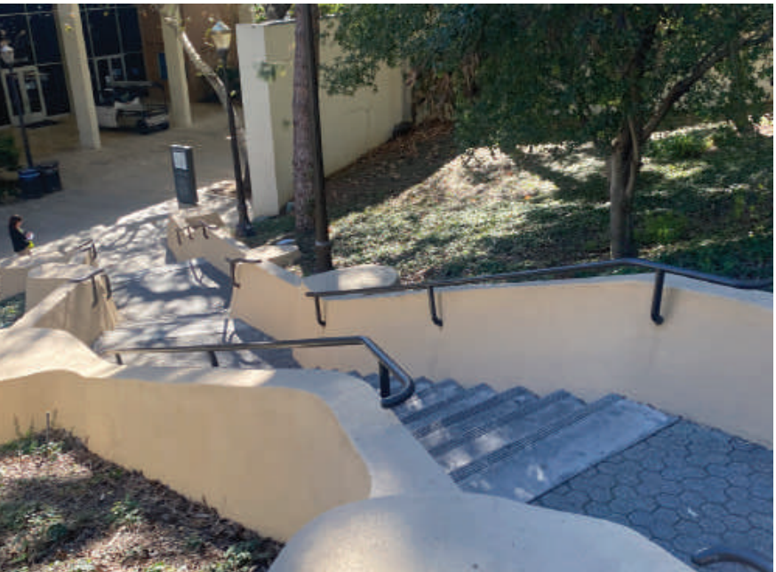
EAST STAIR ENTRANCE
