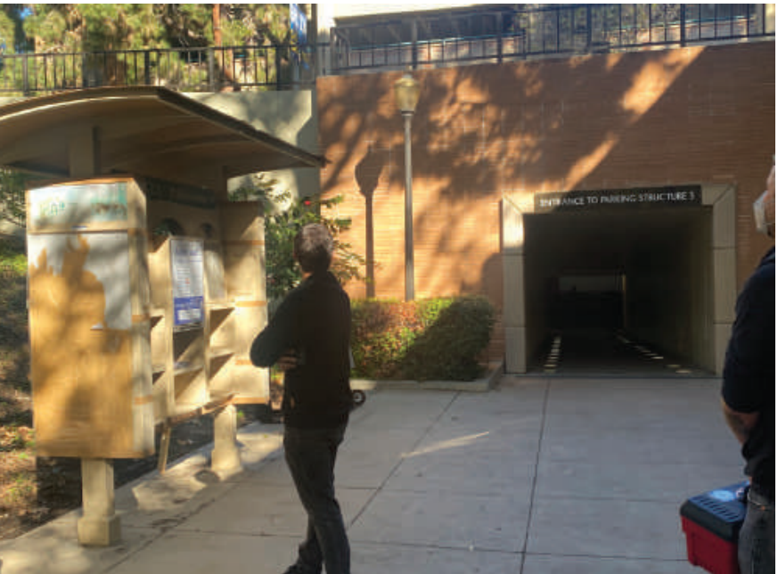
NORTH FACING TUNNEL TO PARKING DECK
