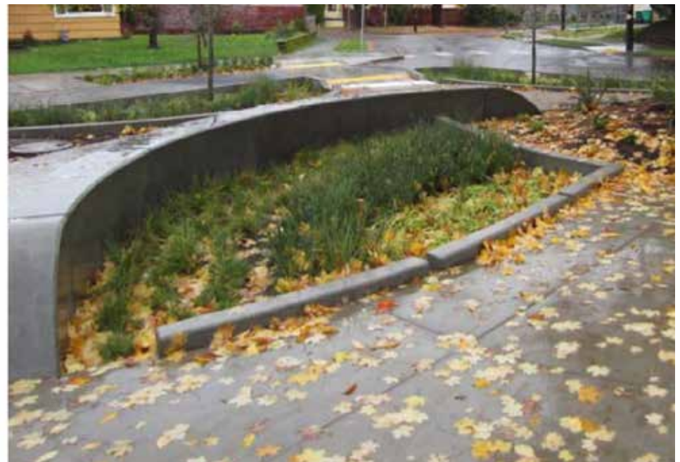
Figure 60: Another images of a stormwater planter combined with a seatwall.
