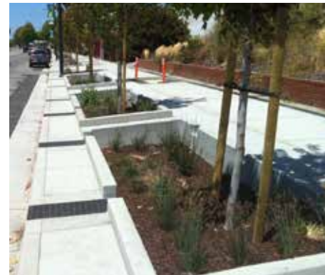
A stormwater infiltration basin can be constructed as part of a sidewalk planter to both increase stormwater capture and create a more pleasant street.
