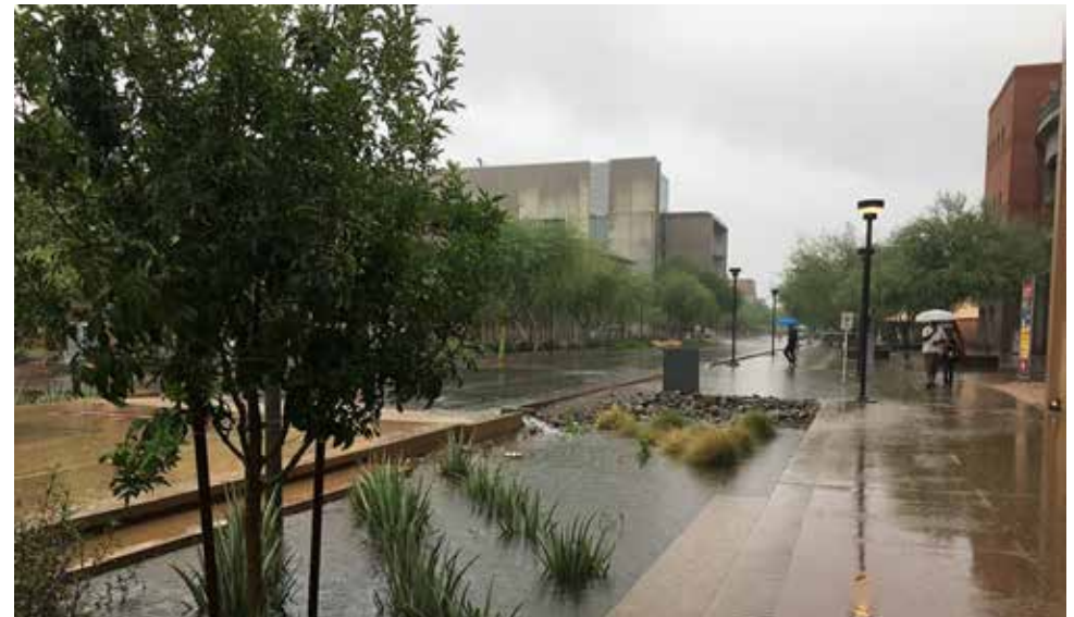
Figure 62: The stormwater planters demonstrated a very high volume for stormwater capture
