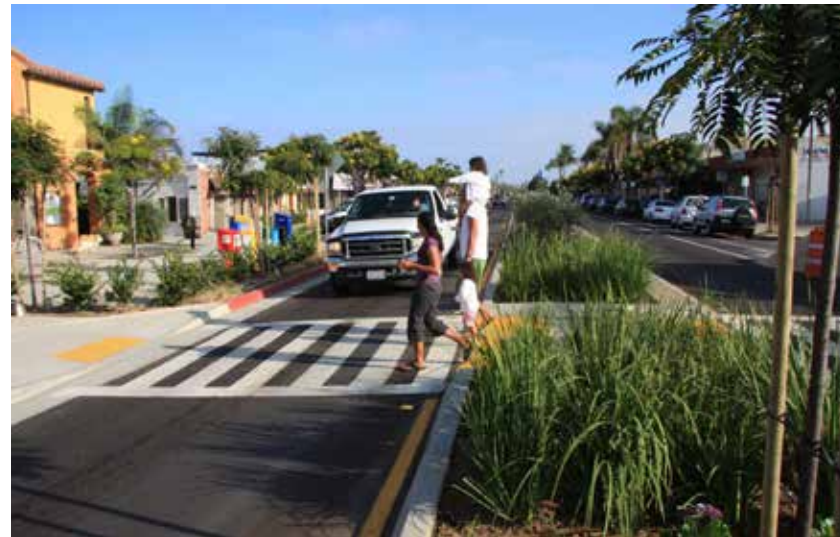
Figure 57: After photo from the median showing shorter cross walks
