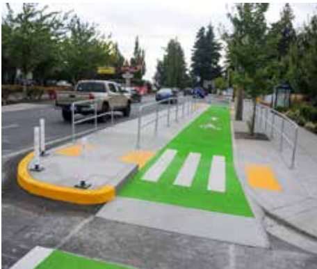
Example of an integrated bus loading zone and protected bike lane, which is recommended in the LA Vision Zero Toolkit
