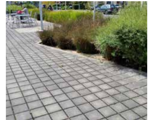
Permeable paving can be used to increase stormwater capture while also beautifying the city .
