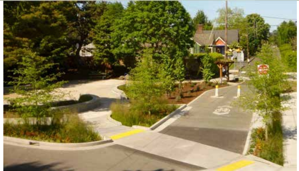
Figure 59: In this photo you can see the new bike lane and stormwater planters.
