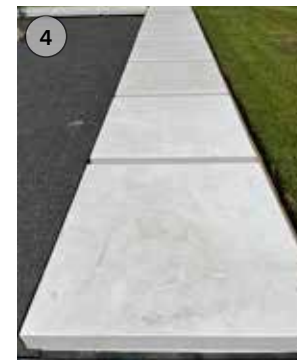
Existing Concrete Seat Wall
