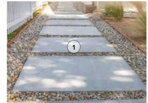
Cast In Place Concrete Pavers with Pea Gravel
