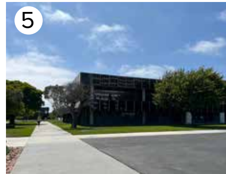
Center Path Looking West
