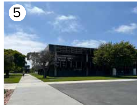
Center Path Looking West
