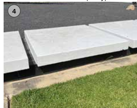
Existing Concrete Seat Wall
